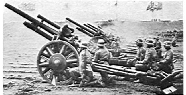
These pieces have the first pattern of pressed steel wheel, but with steel tires rather than rubber ones. In the left picture note the extreme litter of ammunition in the immediate vicinity of the piece; although the uncased projectiles are laid on canvas or paper, they are spotted where much sand and dirt will inevitably be kicked among them. At the right (a battery being fired at the Sportplatz in Berlin before this war) you can get a good idea of tube length, piece silhouette, and pattern of this type wheel.
