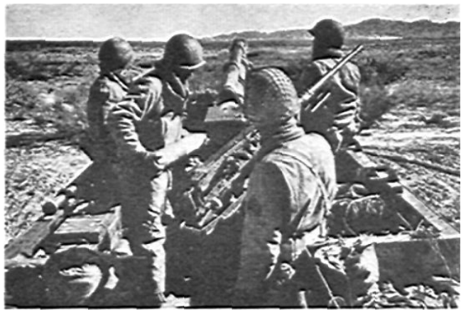
In the early days of Tunisia, half-tracked 105s were used. .50-cal. MG was mounted on a pedestal instead of the ring mount of the M-7. Each carriage had its reel of wire in the right rear corner, and of course personal belongings were lashed all over the outside.
