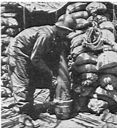
All sand and other dirt must be carefully wiped from each projectile before loading. Note rope grommet to prevent damage to rotating band, and sand-bag ammunition shelter.
