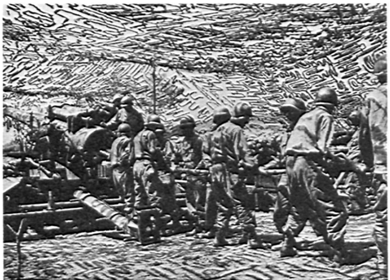
13 cannoneers man the 45-ft. staff to swab the tube after each round. Inverted loading tray is just left of the downward-hinged breech block; to its left is rammerstaff loading bell.
