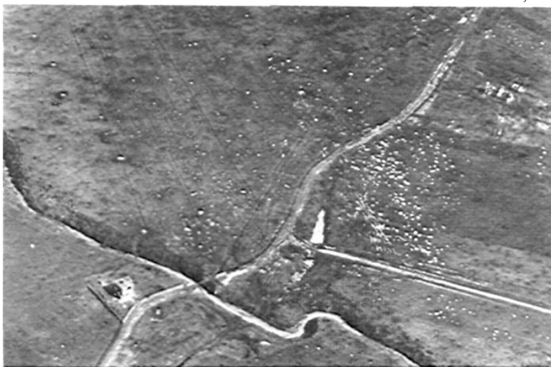
A low-angle oblique of a blown bridge taken from 1,000 ft. This photo was one of many requested by the division engineers; they want to know not only IF a bridge is blown but HOW it is blown. Note reflections from water in innumerable shell holes.
