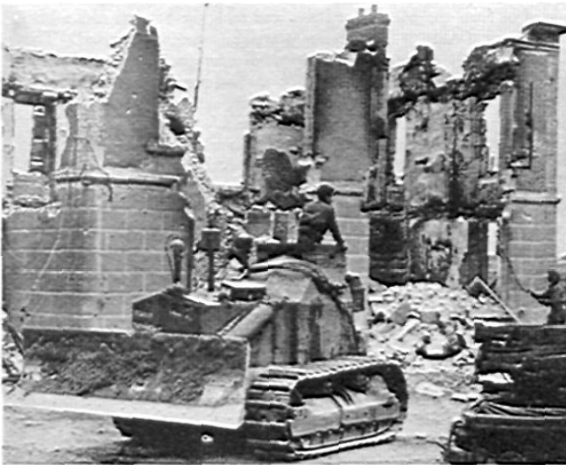
Other towns were badly knocked about, but the armored bulldozer—now apparently 'most as plentiful as the jeep—quickly pushed the debris to one side so that traffic could move without hindrance.
