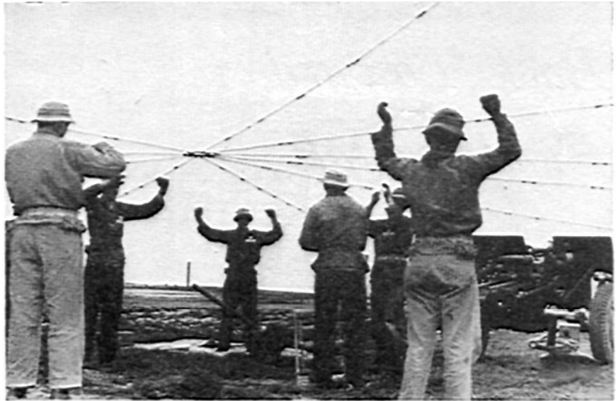
Threading the lacing wire. Note the center ring.
