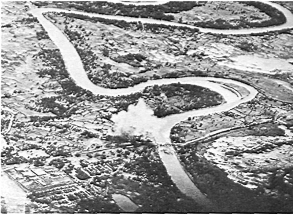
Just south of Mandalay, all rail and vehicular traffic from central and southern Burma to Mandalay, Lashio, and Myitkyina must pass over this bridge at Myitnge. This point has therefore been under steady air attack. Here we see a span knocked out by our Tenth Air Force last January. Since then the bridge has been rebuilt and demolished at least twice. This photo gives a good idea of the open countryside of central Burma, with its meandering Daktawaddi.
