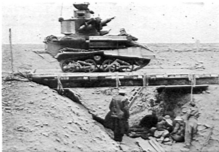
Until they received American equipment, Britain used light tanks like this one in the desert. Small wadis keep engineer troops busy improvising bridges, even in dry weather.
