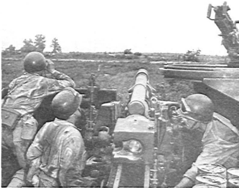
Teamwork blasts the target.—To build a smooth-functioning team, the key men in each M7 are kept together throughout training and are given endless drill, often with service ammunition. Here the section chief, gunner, and No. 1 cannoneer cooperate to lay the howitzer on the target.
