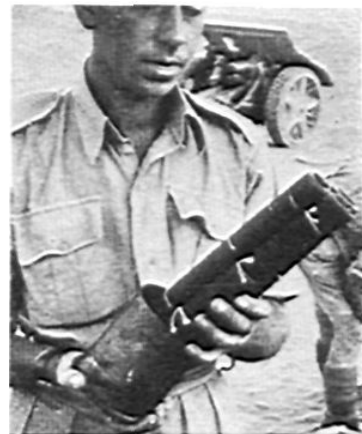
A gunner loads increments for Zone 3 into the reprimed case. Each roll of powder is one zone's increment.
