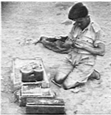
Projectiles and propellants are packed separately. Among the latter, 1 cartridge case is issued per 3 complete charges, primers, and detonators; these are assembled in the field, at the battery position. Projectiles are packed 3 per box, unfuzed; top of the fuze plug is removed for screwing in the upper or top detonator.
