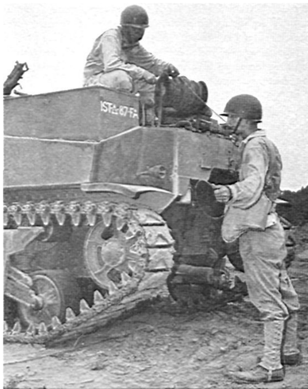
Intra-battery communications.—A reel of wire on the M7 can be unrolled swiftly to provide almost instant communication with the executive's vehicle. The greater dispersion of howitzers in modern armored tactics requires telephone communication where direct voice commands were possible previously, and radio where wire was formerly used.
