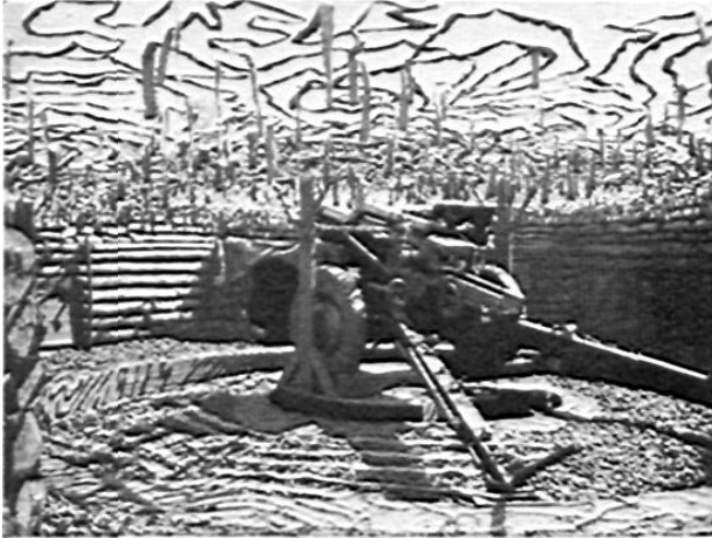
Emplacement "B" has a curbing similar to "A's" for spades, but howitzer itself rests on a turn-table where it is firmly blocked in position.
