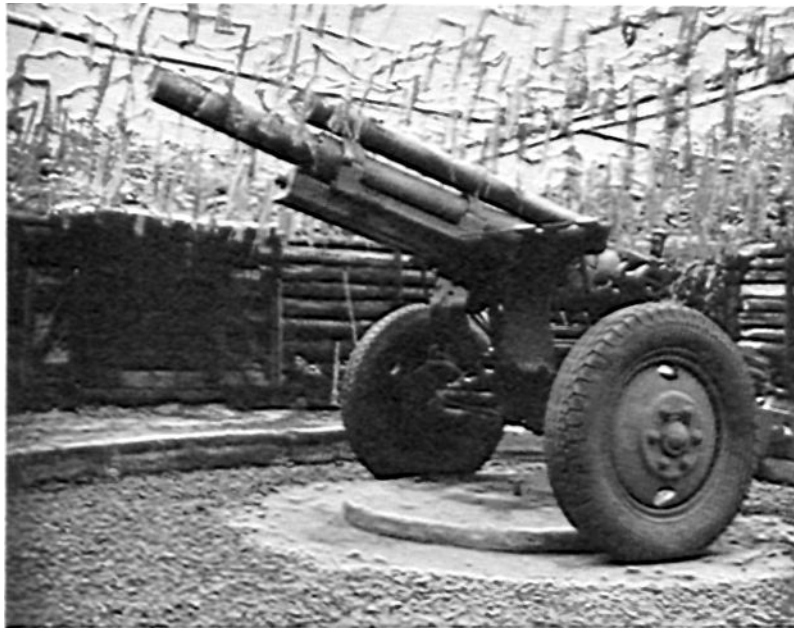
In emplacement "A" the howitzer rotates about a raised disc, to prevent lateral displacement when trails are shifted. Spades fit against circular curbing, to eliminate set-back. Niche for ammunition storage is fitted with hinged "cupboard" doors.
