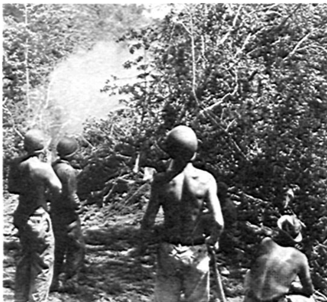
Guadalcanal's draws and gullies were filled with Japanese land mines which had to be tediously detonated by our engineers. Dense growth limits visibility to just a few yards, in the highlands as well as by the coast.
