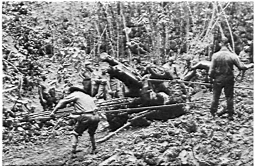
Where New Guinea trails would accommodate a 25-pounder's width, the ground was so rough and grades so steep that block-and-tackle had to be used.
