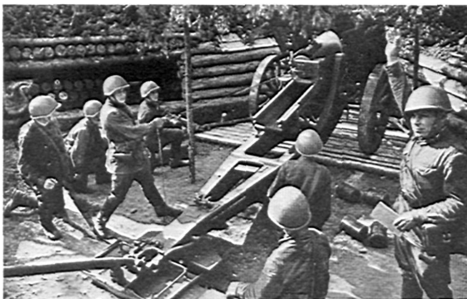
A thoroughly well-organized position! It is dug in, revetted with stout logs, and covered with camouflage net. Wheels of the Russian 15.2-cm. howitzer (M. 09) are on full-width platform for good wet-weather support, and a trail has been dug. Ammunition is carefully yet conveniently stored, with boards between layers; it has weather protection from above, and burlap flaps to keep driving rain away. Cannoneers have smooth footing. Data is chalked on the gunner's side of the shield. The only discordant note is the camouflage-net pole at the left, which would be in the way if the trail had to be shifted very much. The whole thing looks almost like a demonstration set-up—which perhaps it is.
