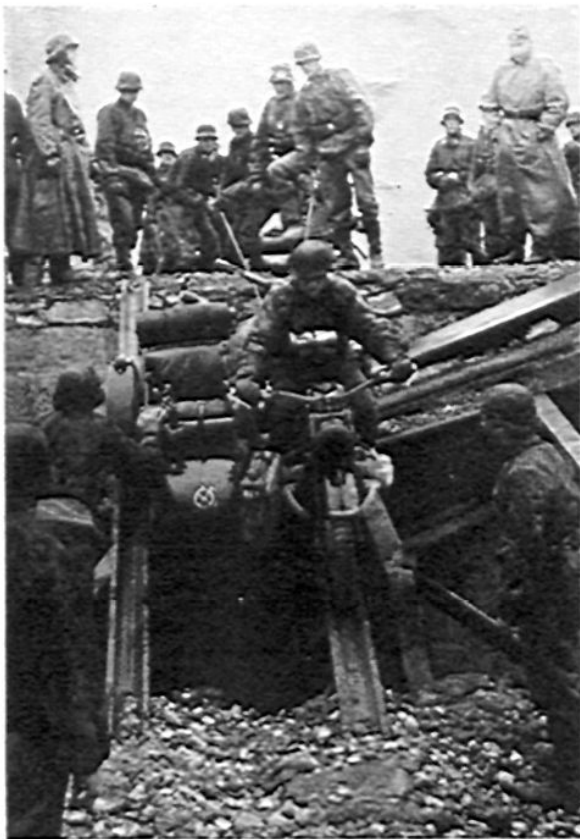
Two lengths of channel iron enable mechanized troops to cross although the bridge has been blasted. (Dever from Black Star)
