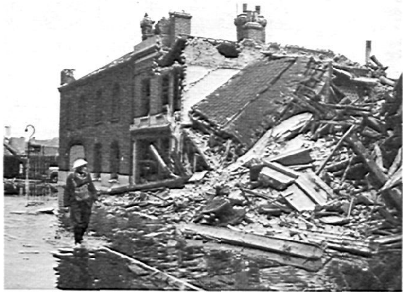
London streets, flooded from hose and broken mains as well as rains.
