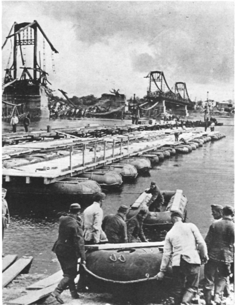
The Russians destroyed some bridges thoroughly, but floating ones rapidly replaced them. (Acme photo.)
