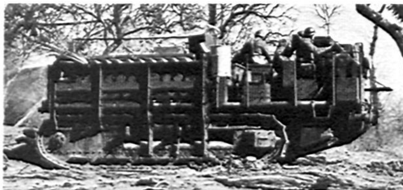
Caisson for the 194-mm. was also a self-propelled, track-laying vehicle.
