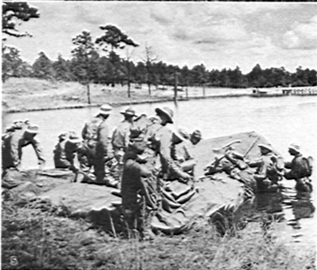
Figure 1—Smooth the tarp and spread on plenty of brush.
