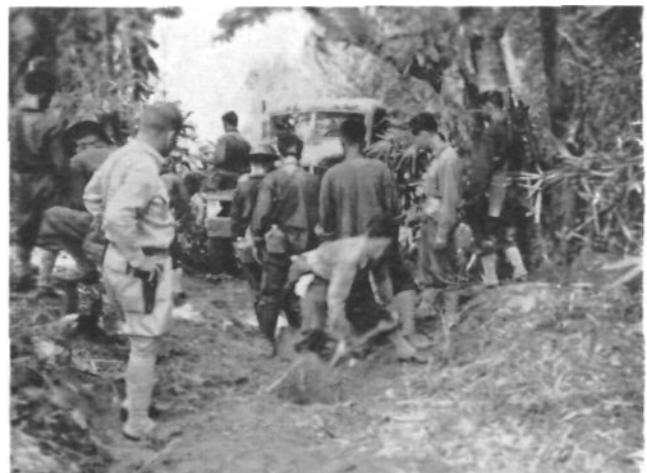
Breaking a road through the jungle
