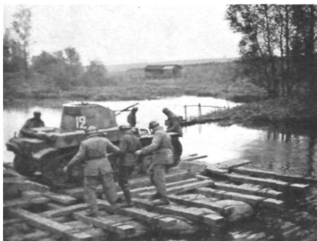
Crossing a river on a raft buoyed by Haber bags filled with straw.
