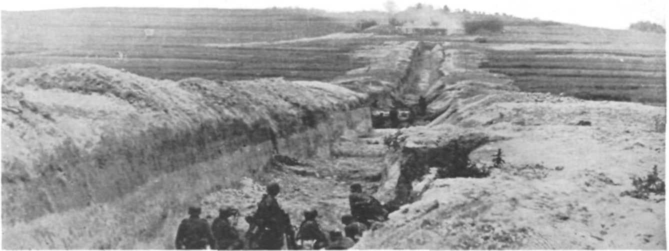
A tank trap constructed at a cost of immense labor by thousands of Russian peasants has been dug hastily across the vast steppes to stop the German Panzers. What happened? The German motorized infantry came up under cover of darkness, took refuge in the ditch, tore down ramps for the tanks to use, meanwhile reducing isolated redoubts by their usual storm-troop methods.
