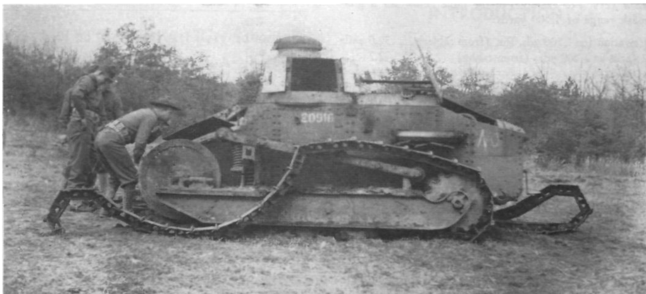
Fig. 10—Effect of mine on Renault tank
