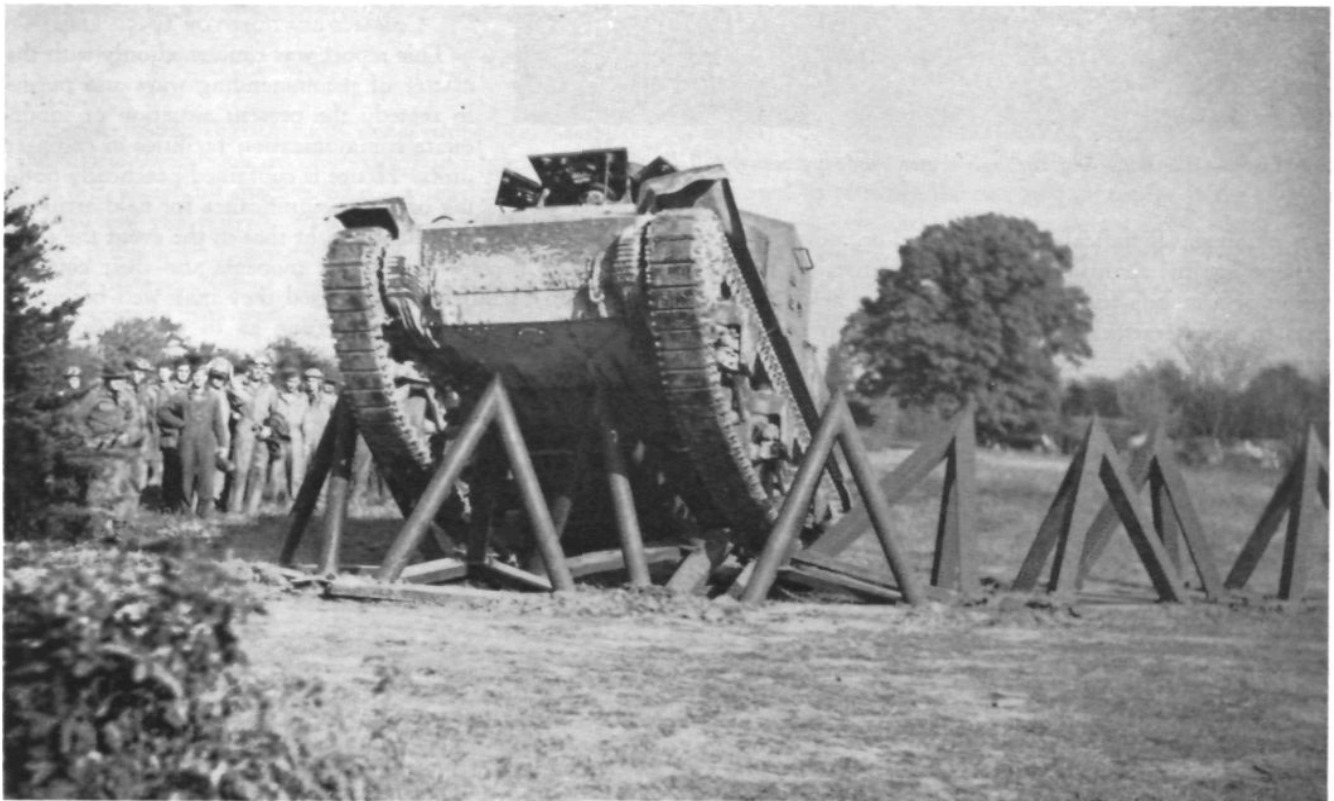
Fig. 6—Tetrahedrons stopping medium tank
