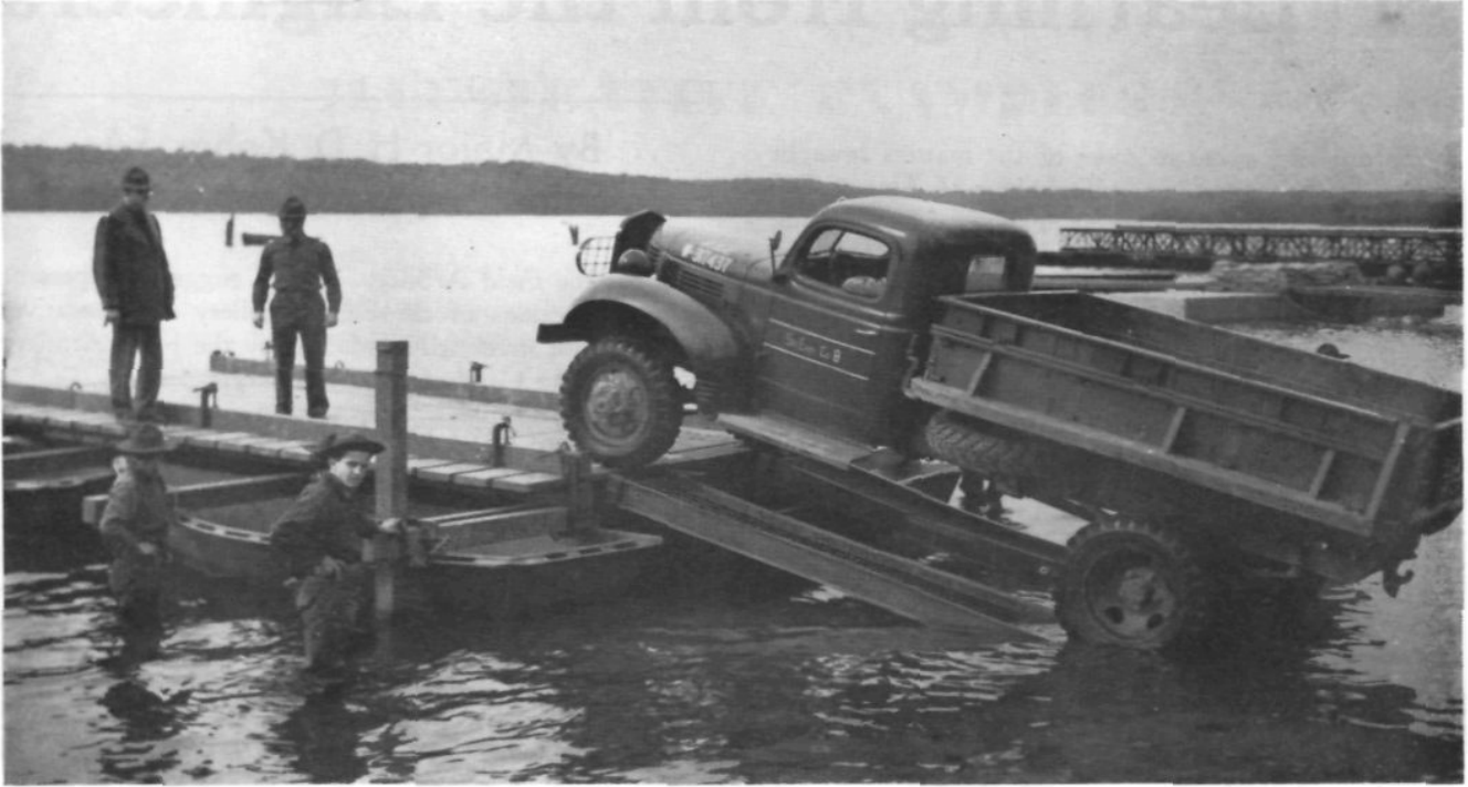
Fig. 2—Assault-boat ferry with girder runways used as ramps
