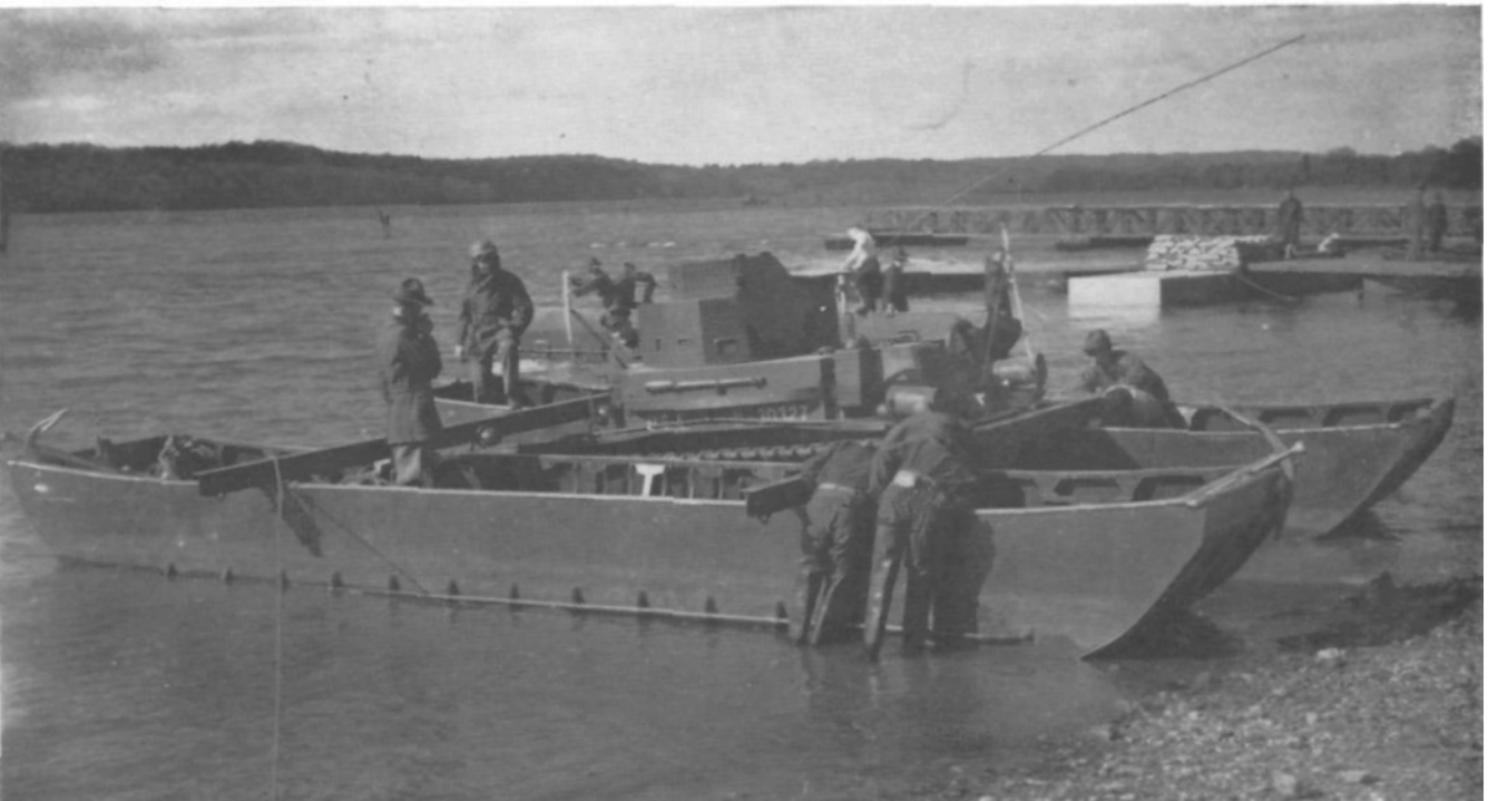
Fig. 3—Tank suspended between pontoons
