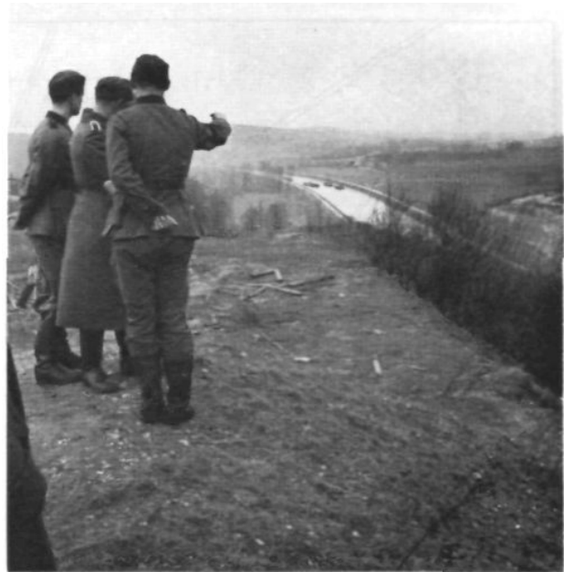
View from northeast corner of the fort, looking down on the Albert Canal at the spot where the pioneers crossed.
