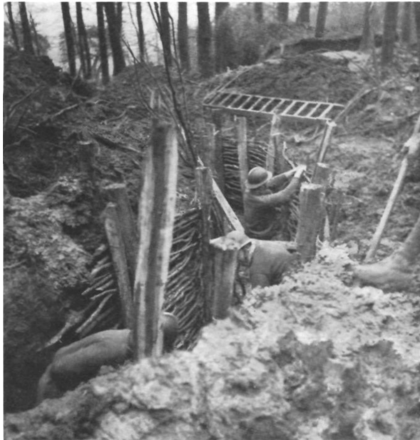
The French trenches were carefully prepared
