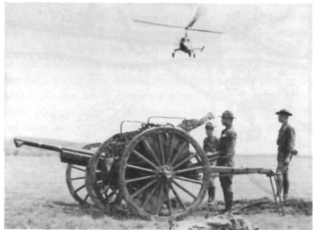
Autogiro hovering near battery
