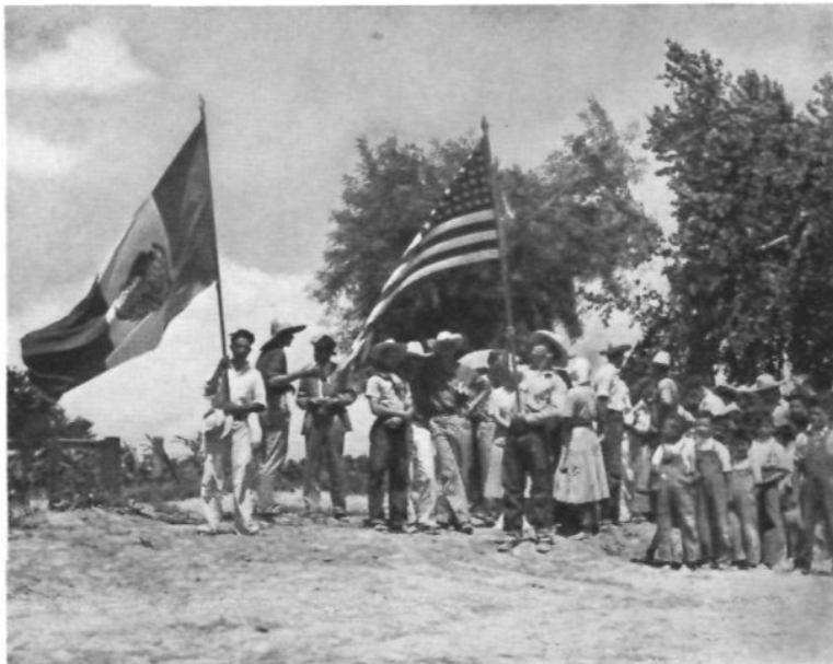
Laying of a cornerstone, July 4th, for a primary school at El Pilar, Torreon, Mexico.
