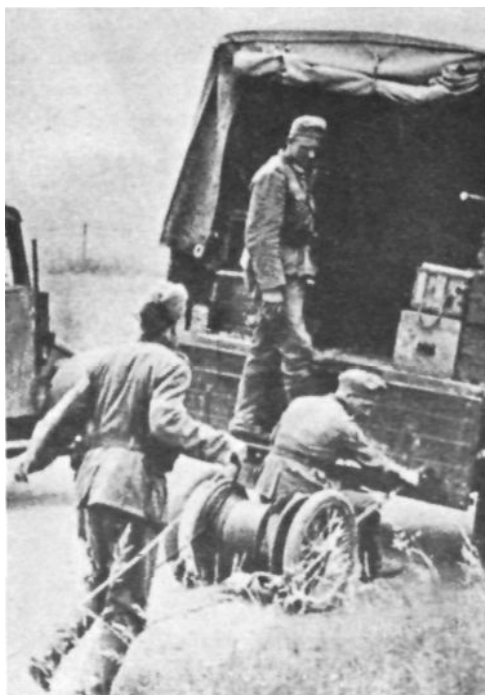
Laying the heavy cable
