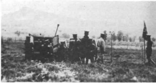
Mexican field artillery (above and in the center). The standard field piece of the Mexican field artillery is 75-mm. St. Chaumond-Mondragon, which has a range of about 5,000 yards. The guns and caissons are drawn by mules. Mexican artillerists practice indirect fire and fire direction in accordance with standard methods, but are inclined to rely on axial methods and direct fire.
