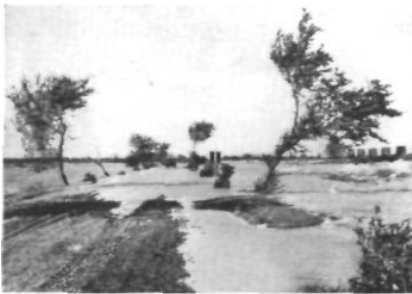
THE ROAD AFTER THE STORM
