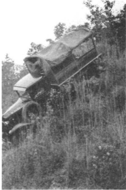
RACKING UP SLOPE WITH PULL-AROUND
