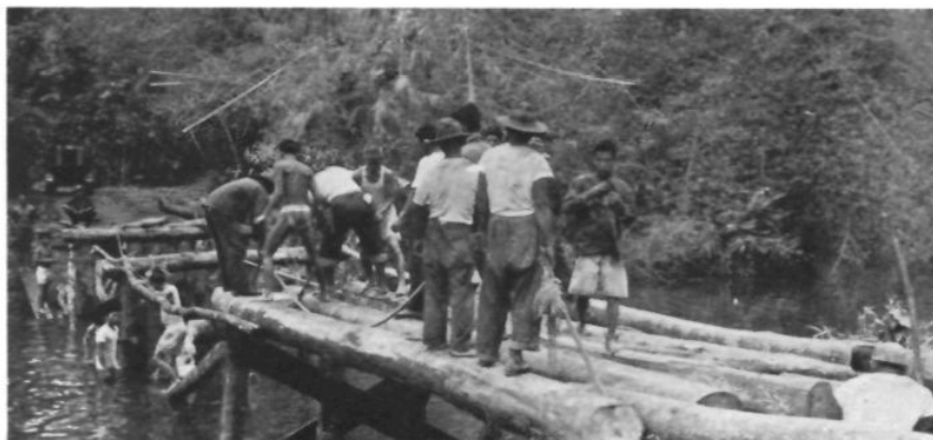
CONSTRUCTION OF A BRIDGE
