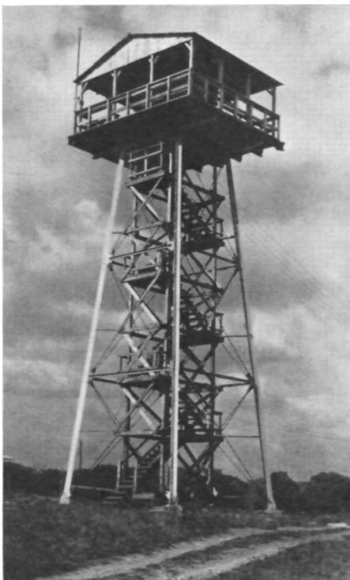
OBSERVATION TOWER FOR CONDUCT OF FIRE.
