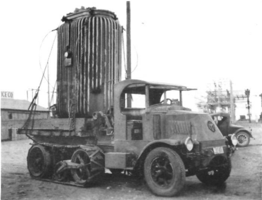
MACK TRUCK WITH HIGH SPEED CRAWLER ATTACHMENT CARRYING A 27,000-POUND TRANSFORMER WHICH WAS HAULED 40 MILES THROUGH THE ARIZONA DESERT
