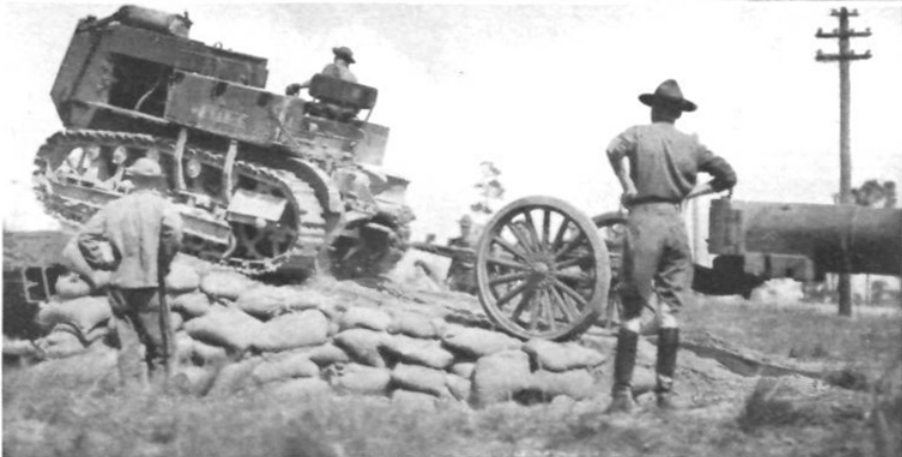
FIG. 4: RAMP MADE ENTIRELY OF SAND BAGS, ABOUT 600 REQUIRED FIG. 5: END FLAT CAR USED AS RAMP FOR 155 GUN FIG. 6: CATERPILLAR HAULING 240-MM. TUBE OVER SAND BAG RAMP
