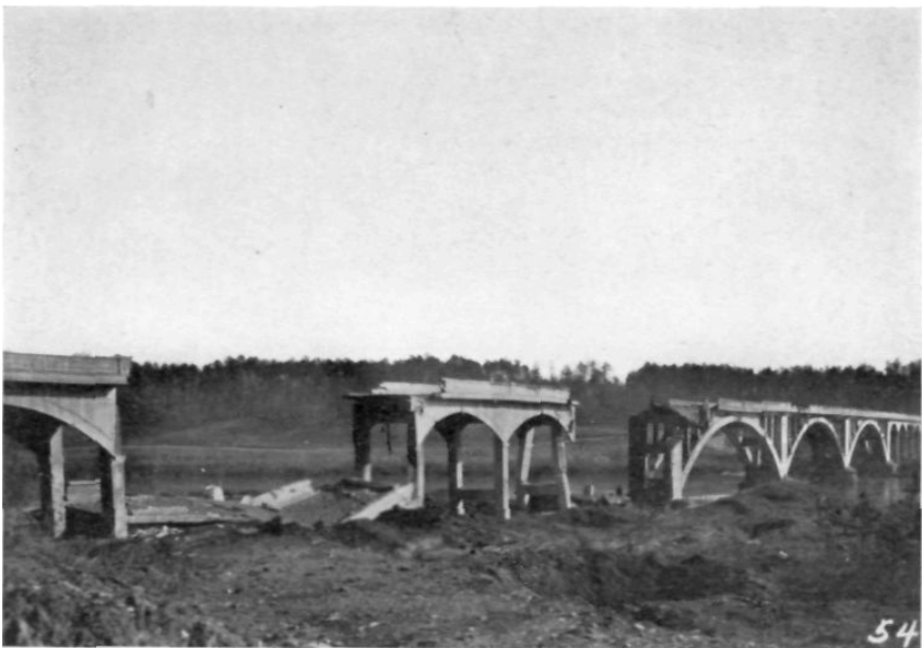
FIG. 2.—BRIDGE AFTER BOMBING AND BEFORE ARTILLERY FIRE
