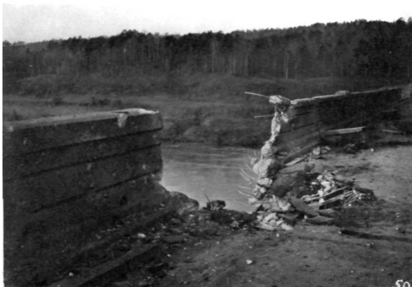
FIG. 5.—EFFECT OF 240-MM. SHELL NO. 11 WHICH STRUCK ON ROADWAY OVER A LONGITUDINAL GIRDER, CUTTING OUT SIX FEET OF THE GIRDER. THIS WAS THE ONLY SHELL THAT APPRECIABLY DAMAGED THE BRIDGE MAIN STRUCTURE
