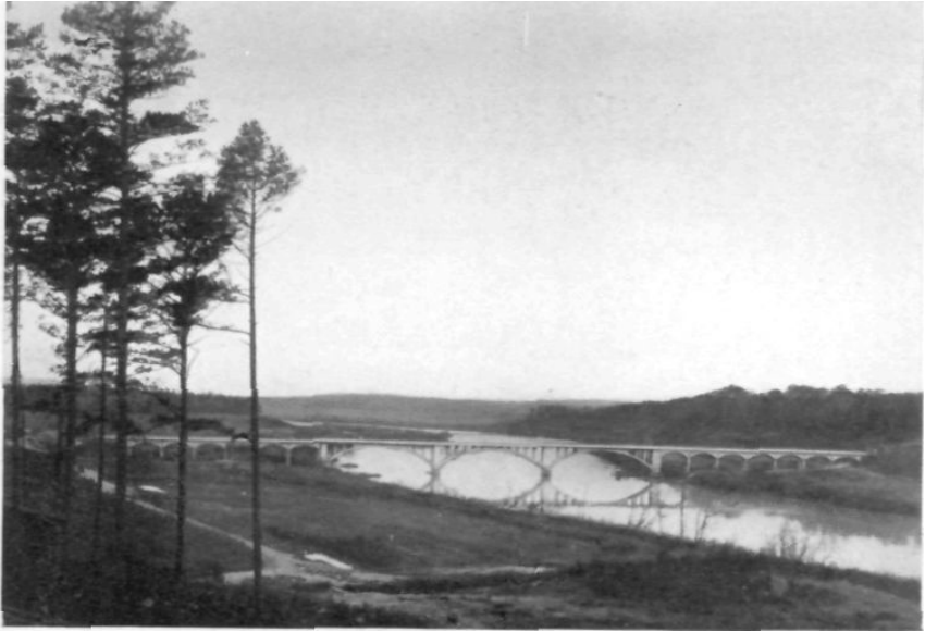
FIG. 1.—VIEW OF OLD BRIDGE BEFORE THE TESTS STARTED. PICTURE TAKEN FROM NEW BRIDGE
