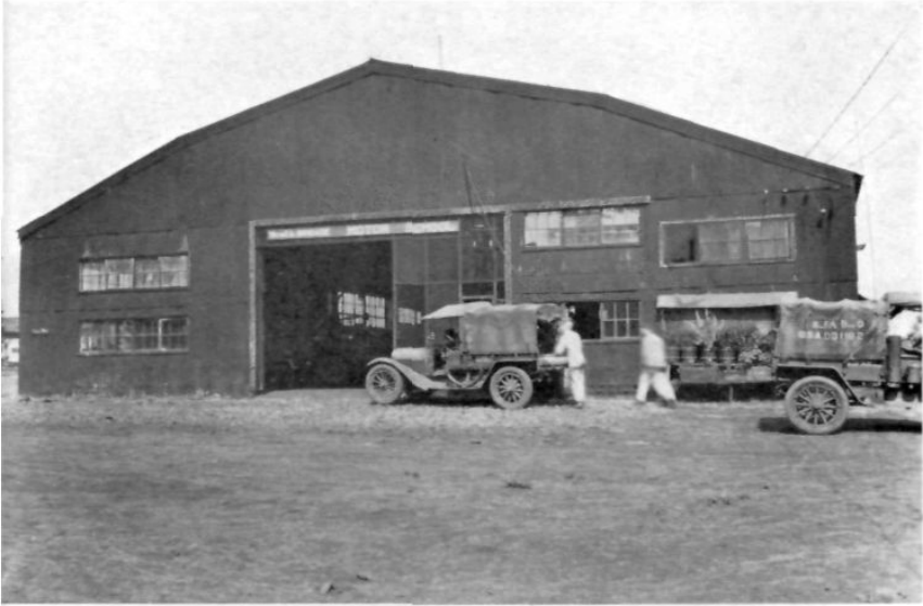
EXTERIOR OF REPAIR SHOP BUILDING, 11TH FIELD ARTILLERY BRIGADE
