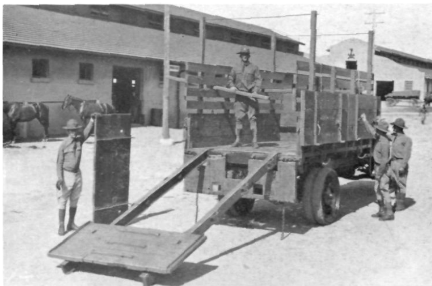
RAMP PARTLY ASSEMBLED. I-BEAMS AND LOWEST SECTION OF FLOOR IN POSITION. ONE SECTION OF PLATFORM BEING HELD TO SHOW UNDER CONSTRUCTION. (NOTE HOOKS AT END OF ANGLE IRONS THAT FIT INTO STRAPS ON I-BEAMS.) TWO SECTIONS OF FLOOR IN CARRYING POSITION ON RIGHT SIDE OF TRUCK
