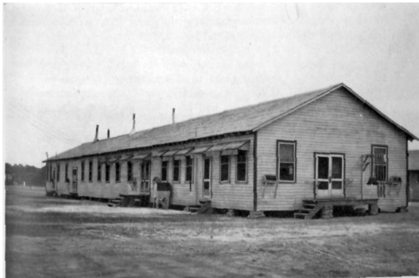
A TWO BATTERY MESS HALL CONSTRUCTED BY 83RD FIELD ARTILLERY.
