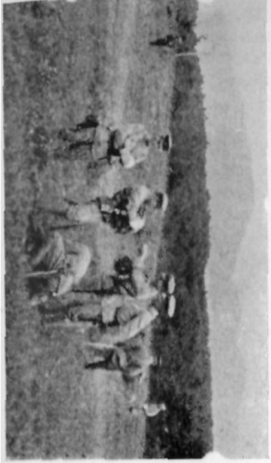
THE BREAST REEL USED EXCLUSIVELY FOR LAYING AND TAKING UP HEAVY WIRE
