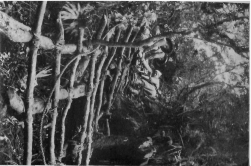
THE THIRD LADDER WAS EIGHTY FEET HIGH, BUILT IN THE FORM OF A DOUBLE SPIRAL IN ORDER TO FOLLOW A CREVICE IN THE ROCK LEDGE
