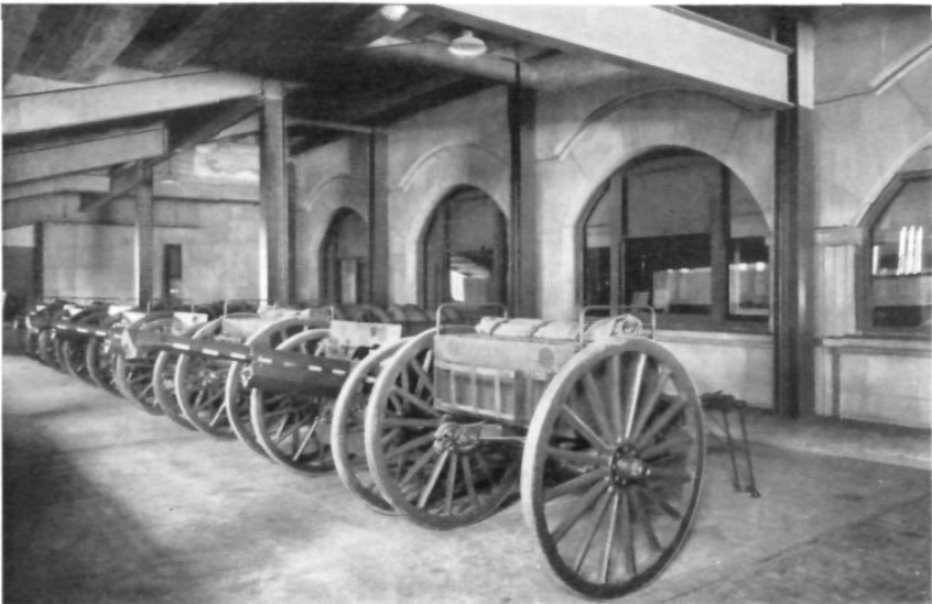
GUN PARK. BENEATH THE VISITORS' BALCONY
