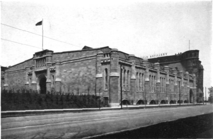
VIEW OF THE ARMORY FROM THE WEST This Shows the New Unit with the Proposed "Memorial Park" in the Foreground.
