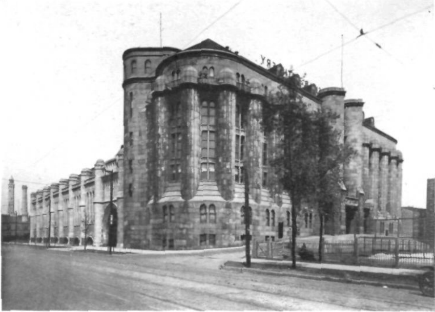
VIEW OF THE ARMORY FROM THE EAST This Shows the First Unit or Administration Section.
