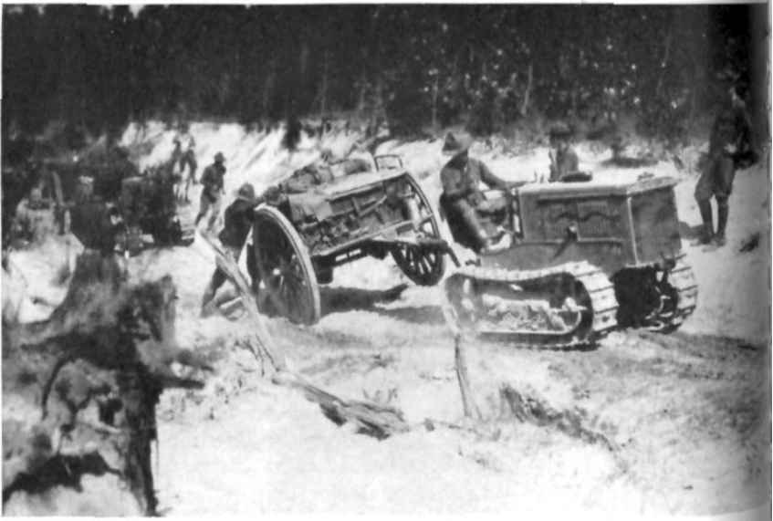
ROUGH GOING ON THE MORGANTOWN ROAD, FORT BRAGG
