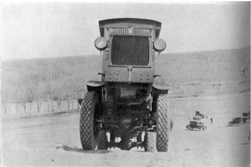
FRONT VIEW OF THE COLEMAN TRUCK REACHING THE TOP OF A GRADE WITH THE LOAD OF CEMENT
