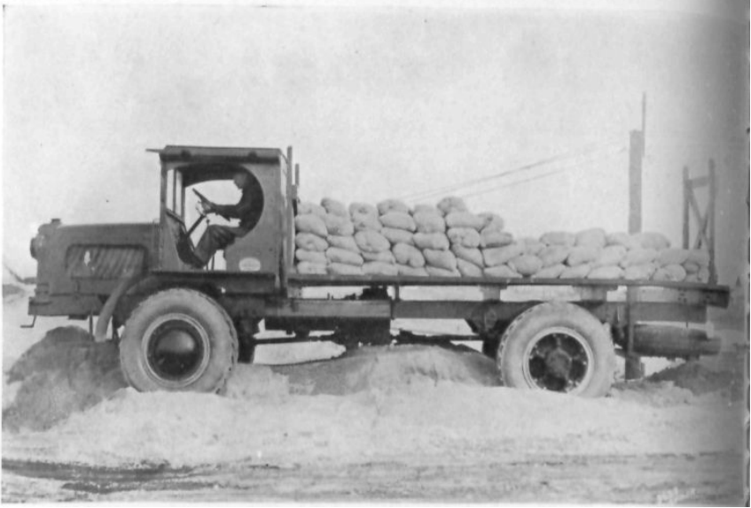
HAULING 10,000 POUNDS OF CEMENT THROUGH LOOSE GRAVEL AND SAND
