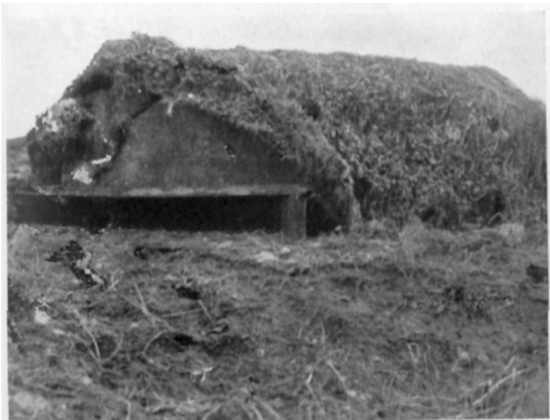
THE PERFECTION FIELD FACILITIES MAY ATTAIN IN A STABILIZED SECTOR Division Observation Post Near Eix.
