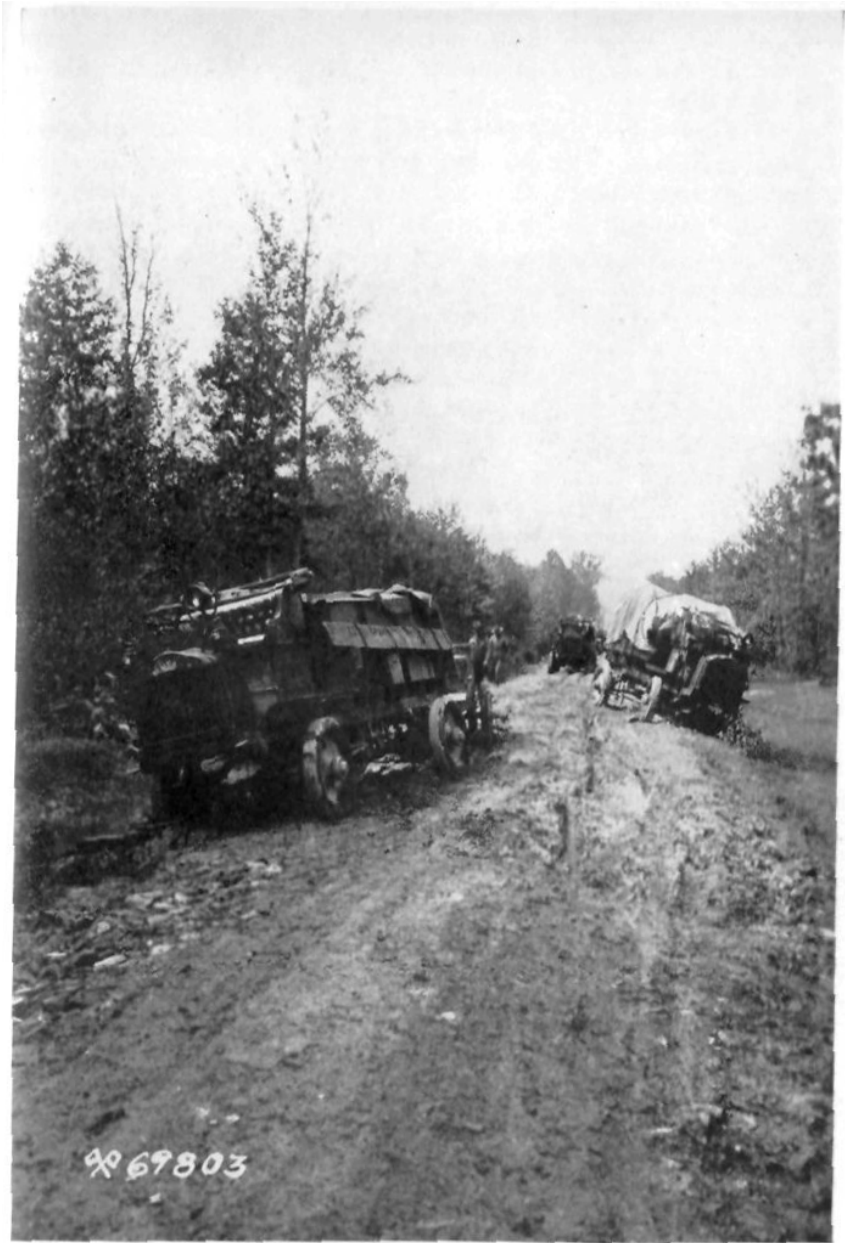
PHOTOGRAPH No. 3.—TRUCKS STALLED FOR LACK OF CHAINS. VERY SLIPPERY CLAY ROAD. QUITE HIGHLY CROWNED.
