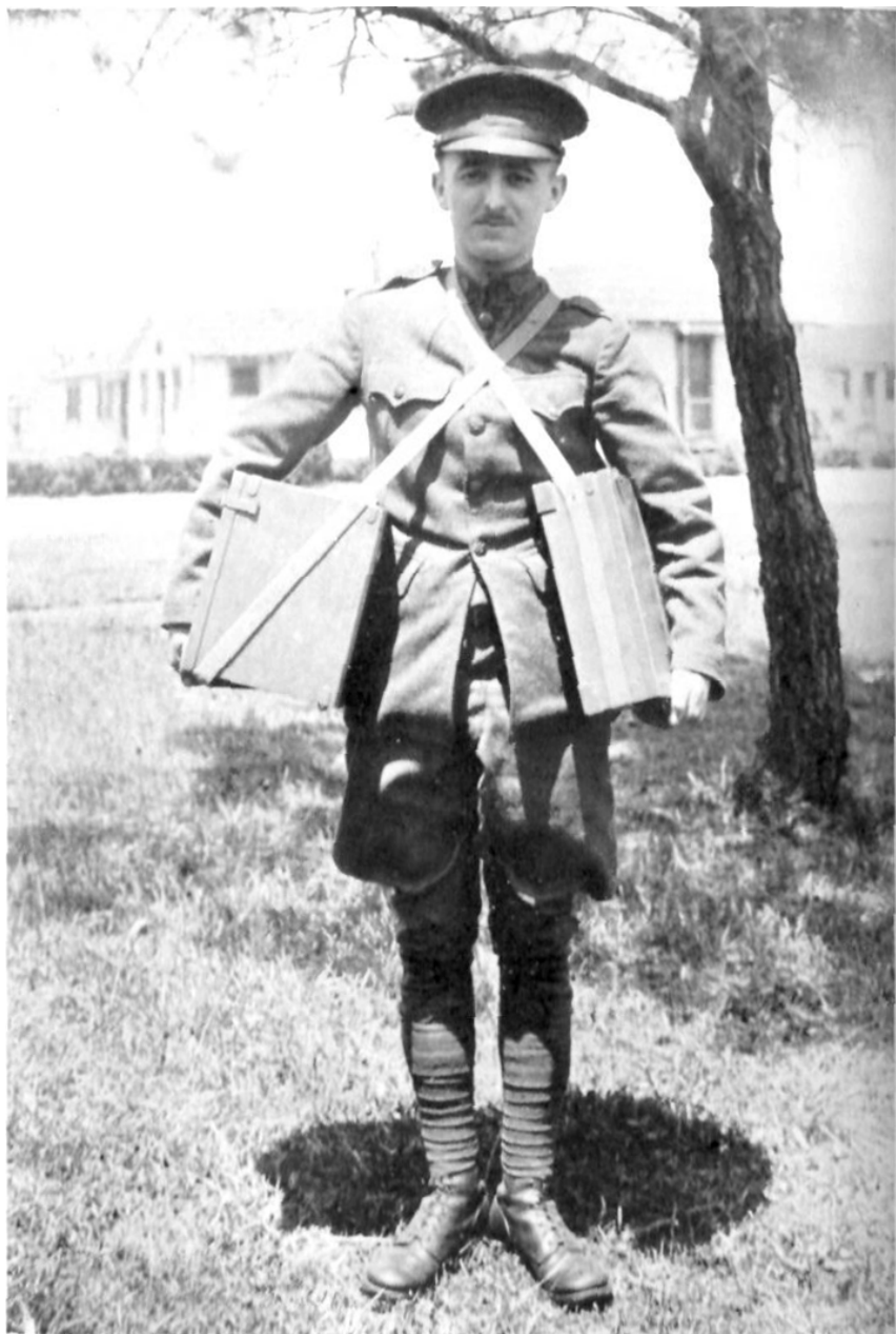
FIG. 4A—SCR-77-A SET. SHOWN AS TO BE CARRIED BY TWO MEN
