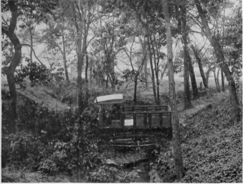
PHOTOGRAPH NO. 3. TRACTOR CAISSON. (See paragraph 4-c.)
