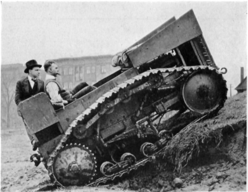
PHOTOGRAPH NO. 14. 2½-TON ARTILLERY TRACTOR MODEL 1920. (See paragraph 8-b.)
