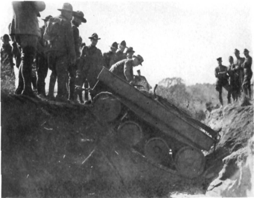
FIG. 4.—RECONNAISSANCE TRACTOR CROSSING A DITCH Block and tackle were used merely to avoid possible accident
