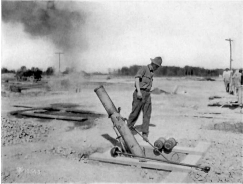
6" TRENCH MORTAR—MARK I—(BRITISH) (NEWTON) SHOWING MORTAR WHICH HAS JUST BEEN FIRED; SHELL; GAS EJECTOR; AND CLINOMETER ATTACHED TO BARREL
