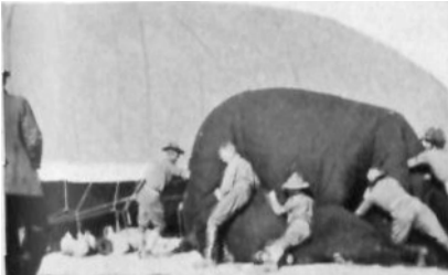
TO WHICH IT WAS ATTACHED BY A PIPE AND THEN THE GAS FORCED INTO THE BALLOON
