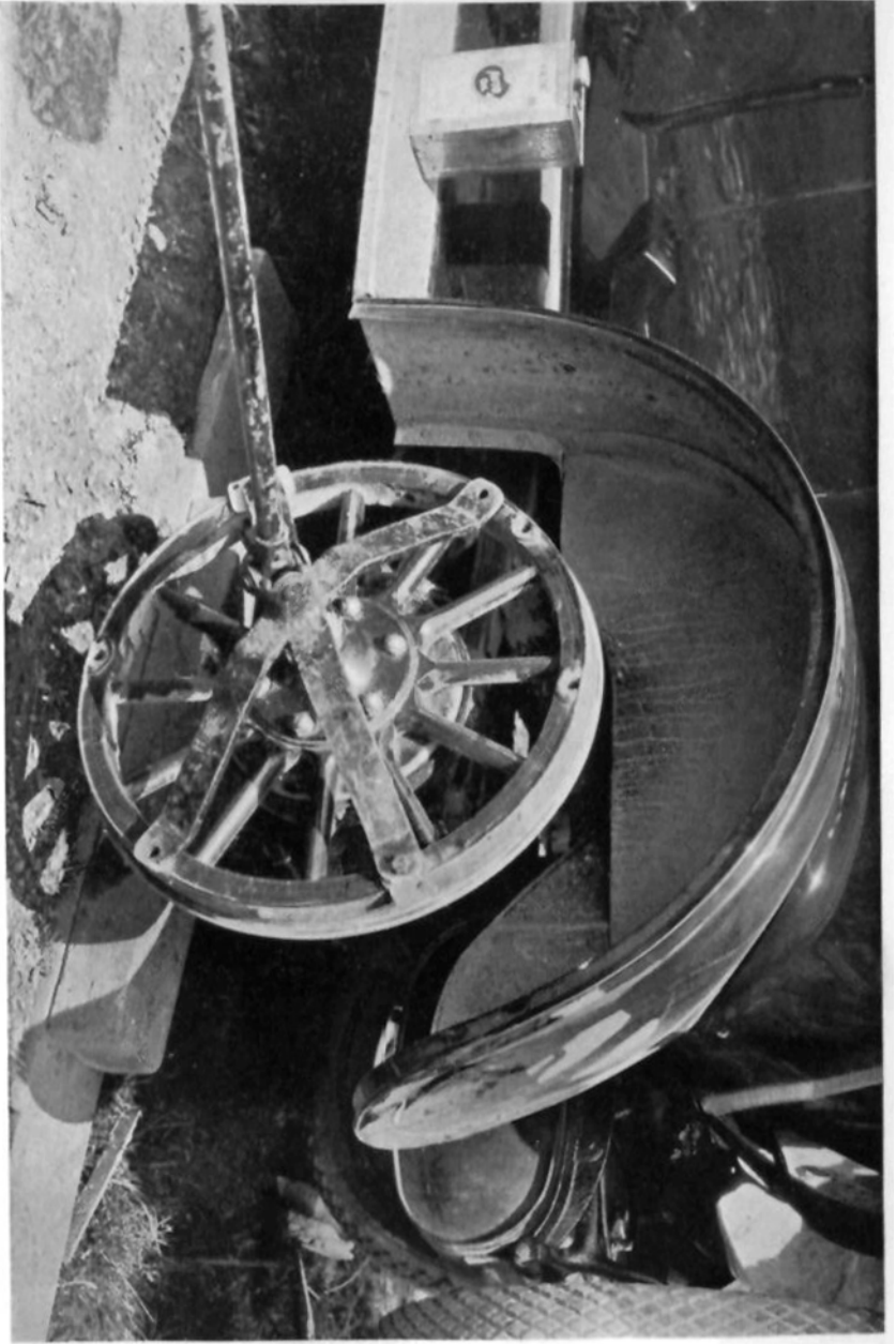
ADAPTATION OF AUTOMOBILE DRIVING WHEEL FOR LOWERING KITE BALLOON
