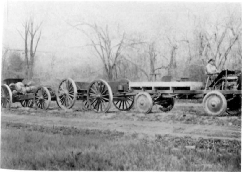
FIG. 8.—A TWO-TON FOUR-WHEEL DRIVE TYPE TRUCK PULLING SECTION OF SIX-INCH HOWITZER MATERIEL ON THE ROCK TESTING ROAD AT ROCK ISLAND ARSENAL.
