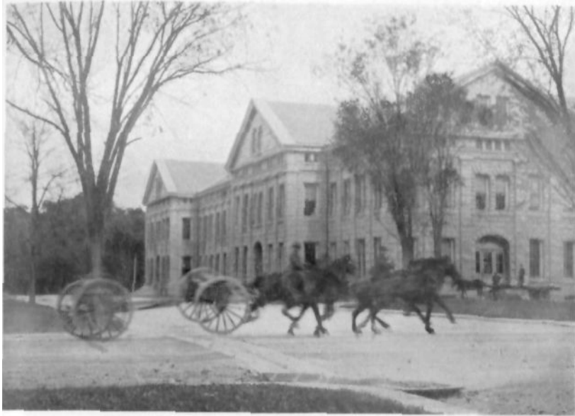
FIG. 11.—RAPID TOWING WITH AN AUTO TRUCK WILL BREAK UP RIGID VEHICLES MUCH MORE QUICKLY THAN HORSES CAN DO AT THEIR WORST. THE CROSSING THE LIMBER HAS JUST STRUCK DOES NOT PROJECT MORE THAN TWO INCHES ABOVE THE ROADWAY. IT IS A BARELY NOTICEABLE OBSTRUCTION.
