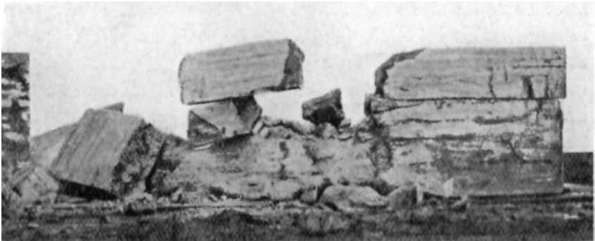
THE SAME WALL AFTER SEVERAL SHOTS
