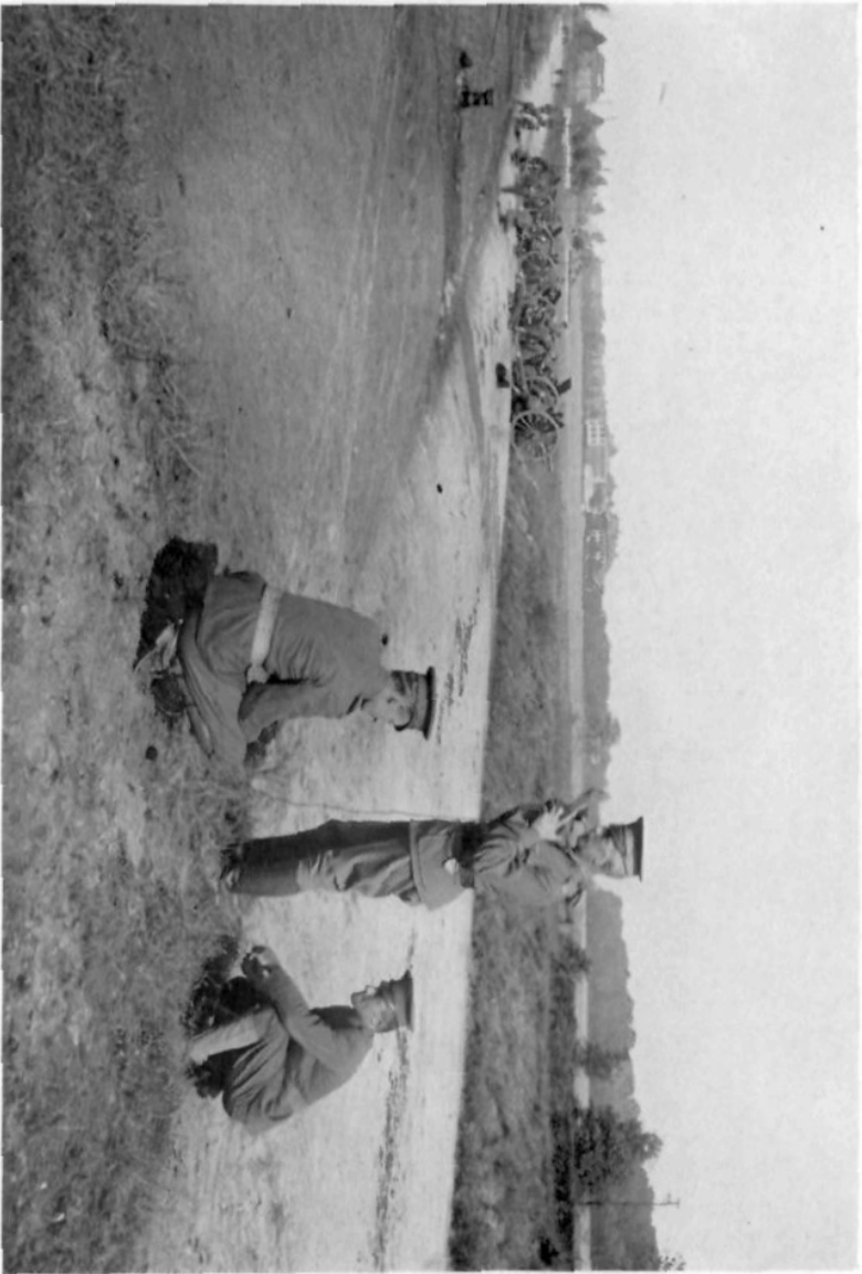
TEST OF LOUD SPEAKING TELEPHONE AT FORT MYER, VA. THE ILLUSTRATION SHOWS THE USE OF THE TELEPHONE BY THE BATTERY COMMANDER WITHOUT INTERVENTION OF OPERATORS
