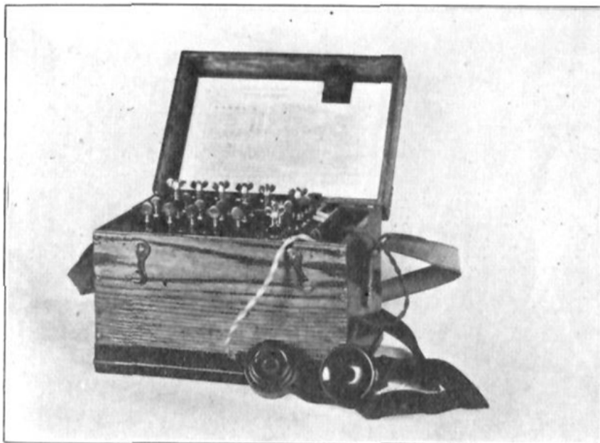
THE FIELD SWITCH BOARD
