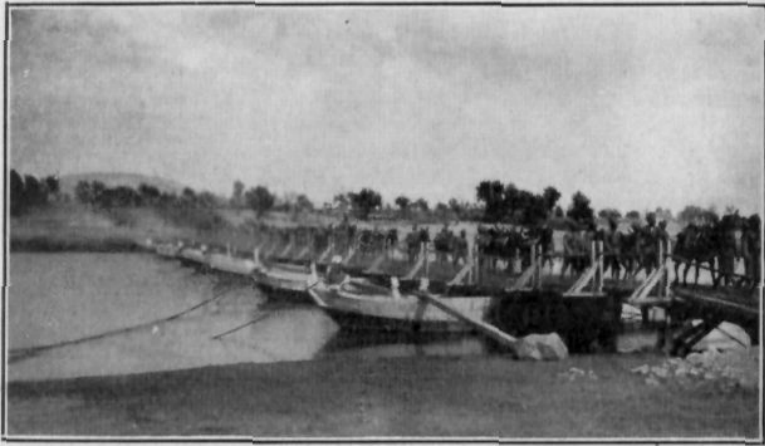
MOUNTAIN BATTERY CROSSING PONTOON BRIDGE OVER KABUL RIVER.
