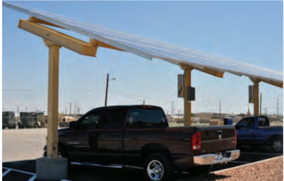
Solar panels used as carports at Fort Bliss, Texas. (Photo by Samantha Reho)
