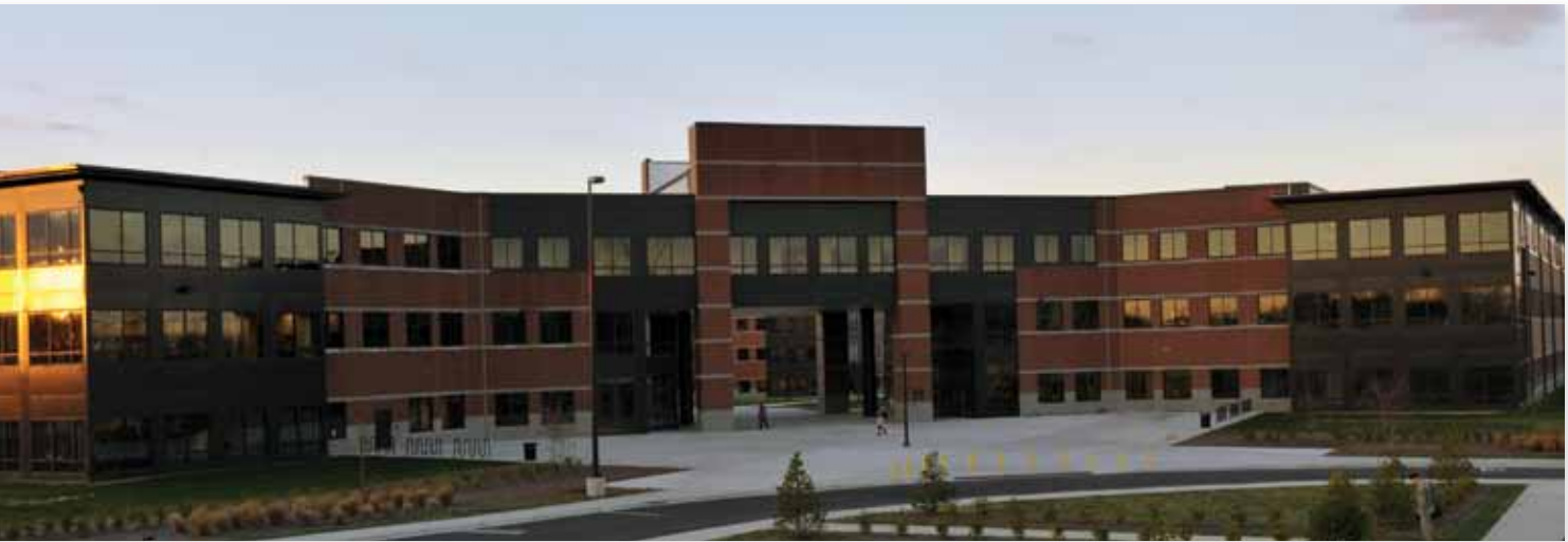
The LTG Timothy J. Maude Complex is the largest administrative center in Kentucky at more than 883,000 square feet. The complex opened May 27, 2010 and is home to Army Accessions Command and Army Human Resources Command.
