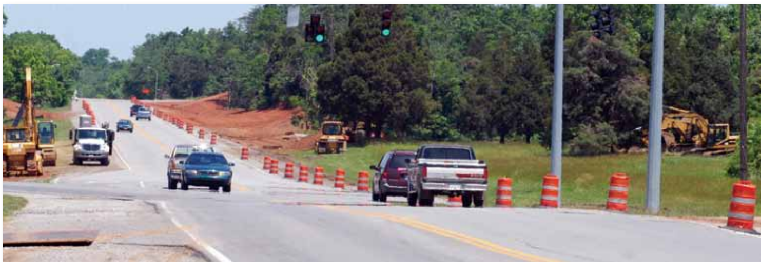
Most of Wilson Road on Fort Knox was widened from two to four lanes because, with its proximity to the newly constructed LTG Timothy J. Maude Complex, which houses up to 4,400 workers, it became one of the post's main thoroughfares.
