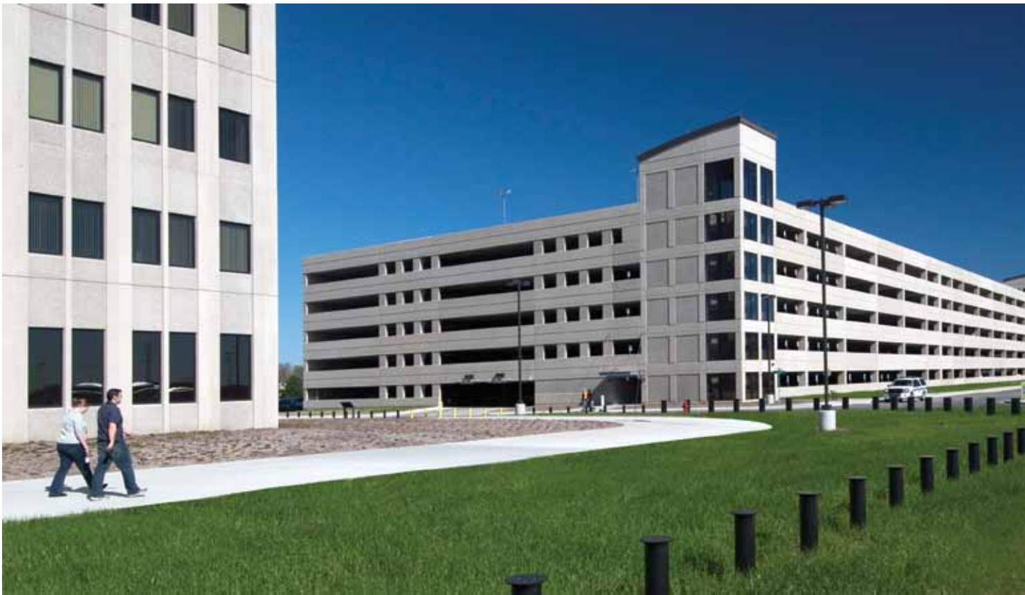
The new parking garage that was constructed in conjunction with the new BRAC administrative building. Cooperation between the architects, builder and U.S. Army Garrison - Detroit Arsenal public works engineers enabled the building to be completed six months ahead of schedule.
