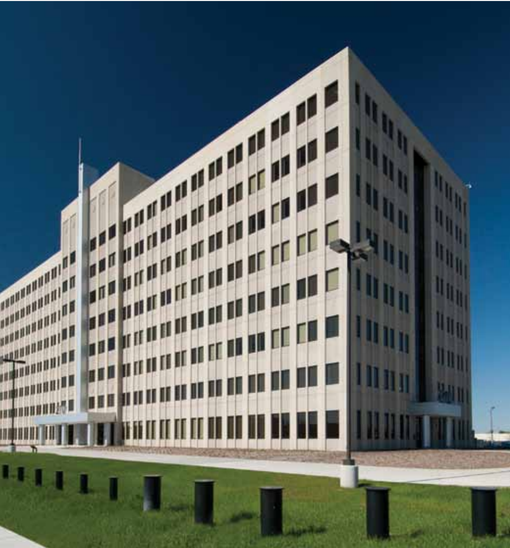
The LEED Silver BRAC administrative building at the U.S. Army Garrison - Detroit Arsenal was completed nearly $30 million under budget, cost overruns were kept to less than two percent and the building was completed three months ahead of schedule.
