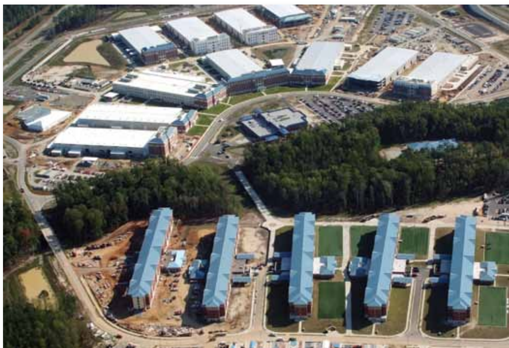
The Army's new Ordnance School campus is located north across Route 36 from the main portion of the Fort Lee installation, significantly increasing the footprint of the post's training facilities. (U.S. Army photo by Albert Cruz)
