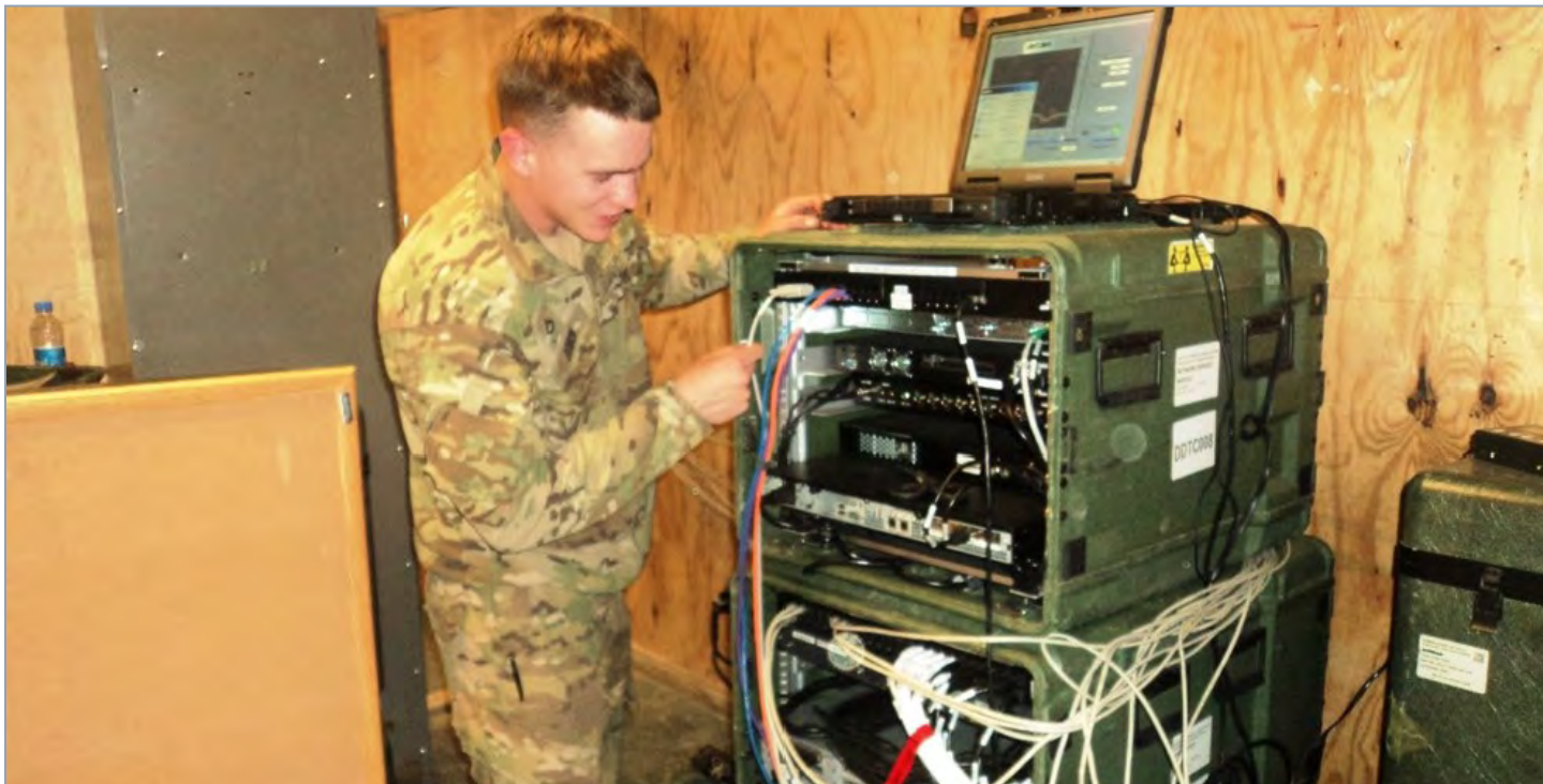
SPC Tony Jobin conducting initial setup of the new DDTC system
